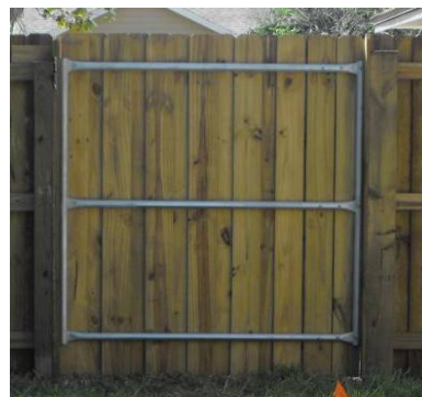
Steel Gate frame
